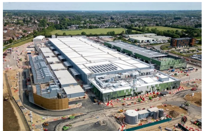
Google's new data centre under construction in Hertfordshire. © BBC
